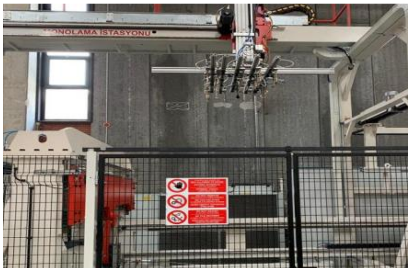
FIGURE 9: THERMOFORMING PRODUCTION LINE
