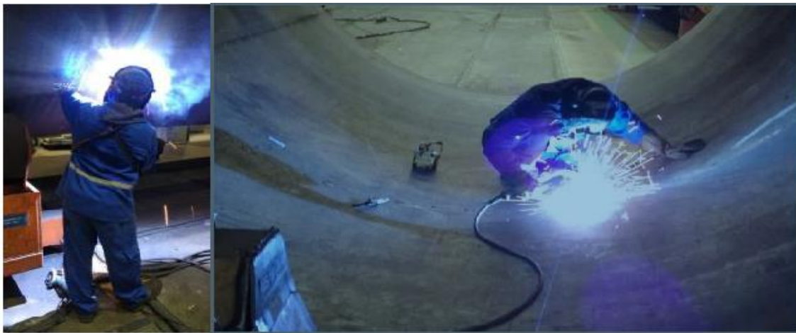
FIGURE 24. THE TIME NEEDED TO REPAIR A SECTION WITH A REFERENCE LENGTH OF 1 M AND 20 MM DEPTH IS ESTIMATED TO BE BETWEEN 6-12 HOURS IN GRI USE CASE
